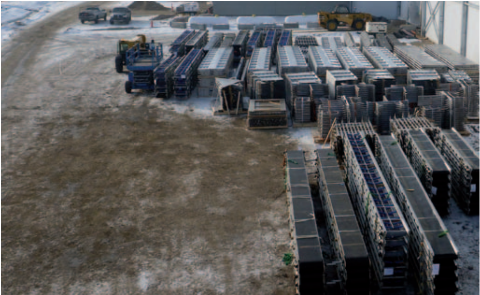
December 2012 | Start of installation Dezember 2012 | Montagebeginn
