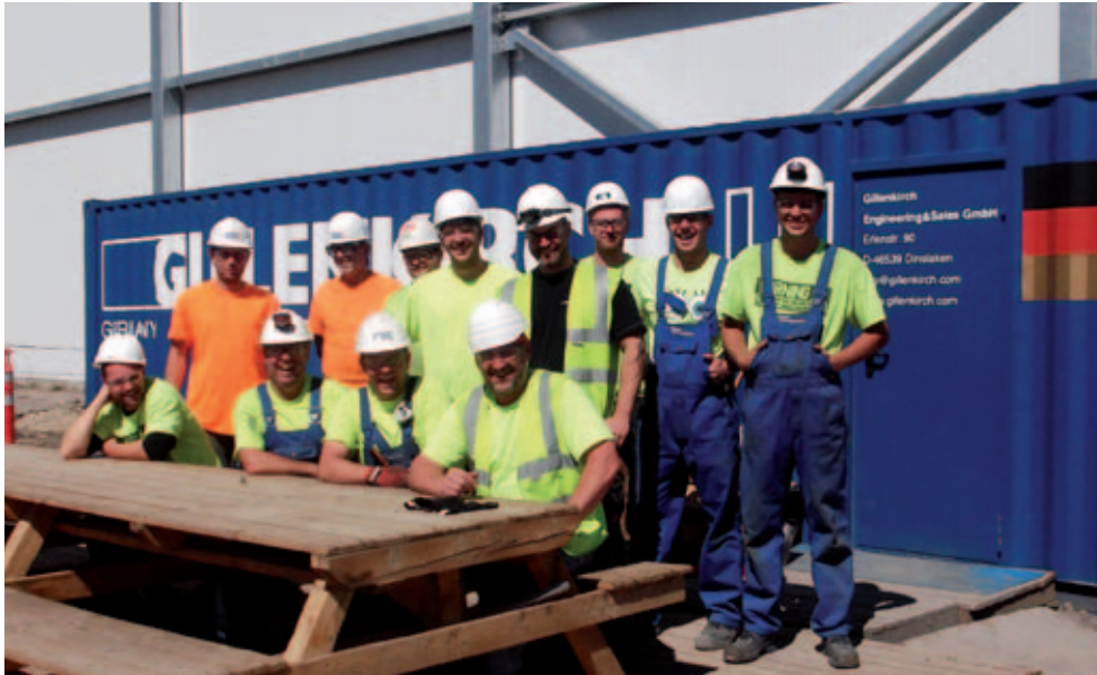
Installation team | Gillenkirch | Fresh Link | Mager Electrical Engineering Montageteam | Gillenkirch | Fresh Link | Mager Elektrotechnik
